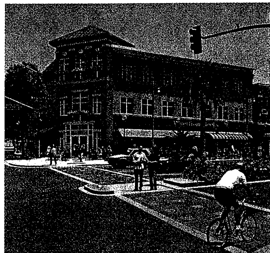
Figure 3.C.45: The corner of Georgia Street and Mare Island Way should offer a dynamic and lively place that attracts people
