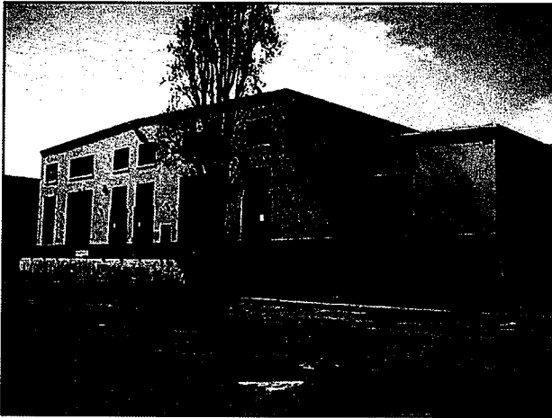
M – Masonry Industrial Shops (Building 0461)
