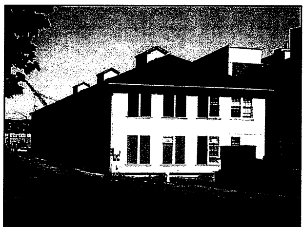
R – Metal-Clad Administrative, Institutional, Or Commercial (Building 0208)
