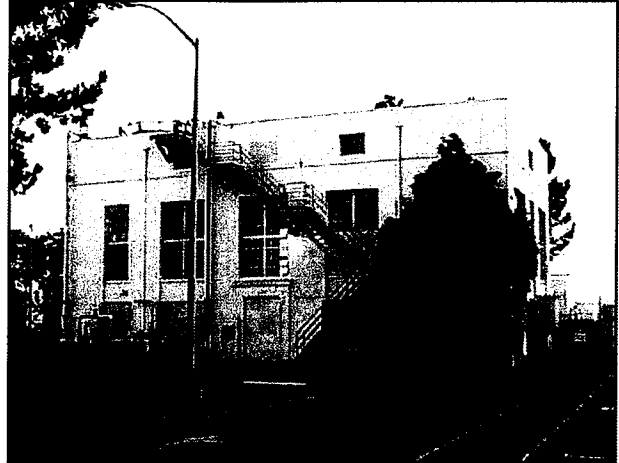
H – Other Infrastructure (Building H074)
