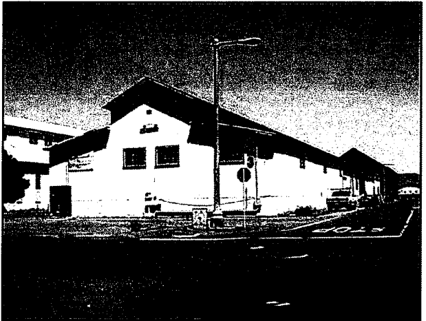
L – Metal-Clad Industrial/ Ordinance Storage Or Warehouse (Building 0223)
