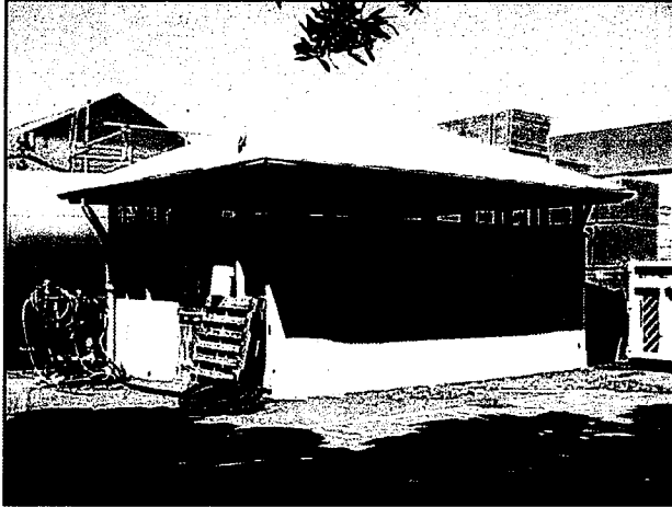
G – Latrine (Building 0077A)
