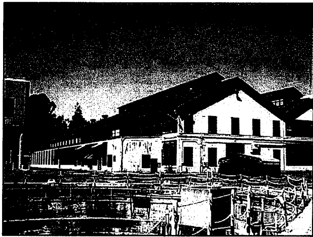
O – Metal-Clad Industrial Shops (Building 0116)
