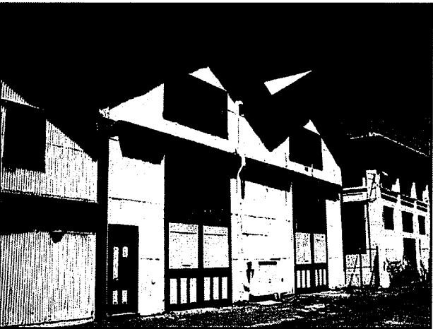
K – Wooden Industrial/ Ordinance Storage Or Warehouse (Building 0111)
