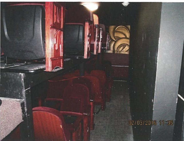
Item 31: Storage area beneath extended stage – fair.
