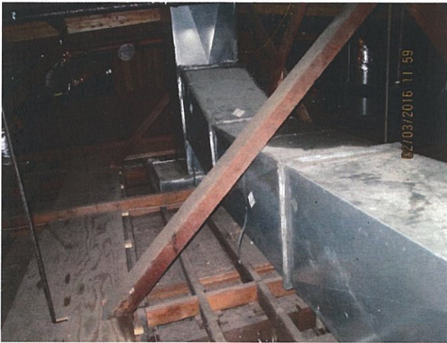
Item 36F: New ductwork to rooftop units – good.
