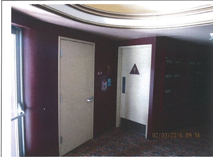
Item 11B: Corridor to left of lobby – fair.
