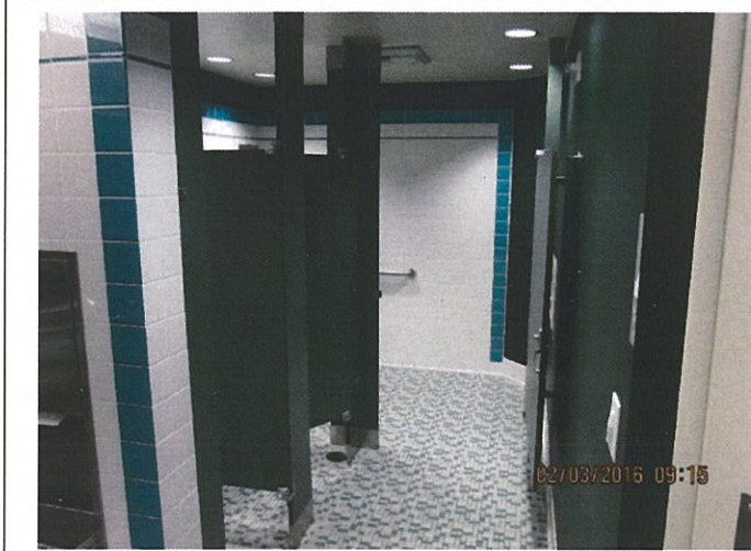
Item 16B: Restroom partitions – good.
