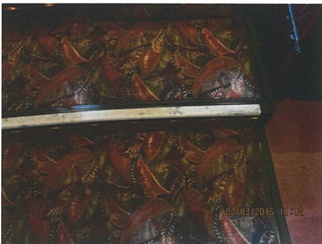
Item 18C: Stair nosing.
