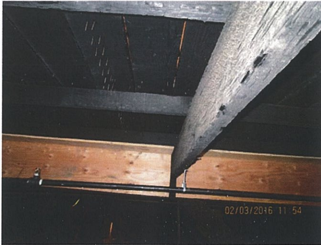
Item 36E: Reinforced beam.
