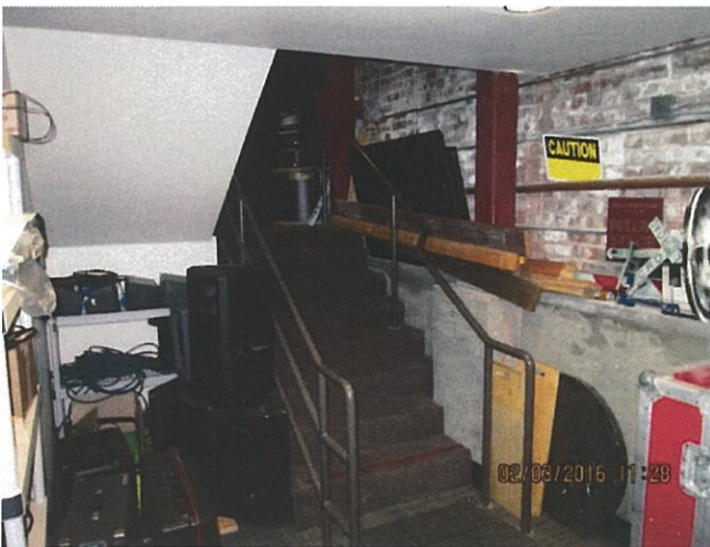
Item 27: Stairs from storage up to stage.
