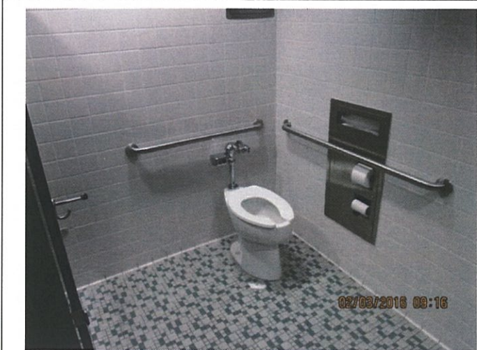
Item 16C: Restroom stalls – good.
