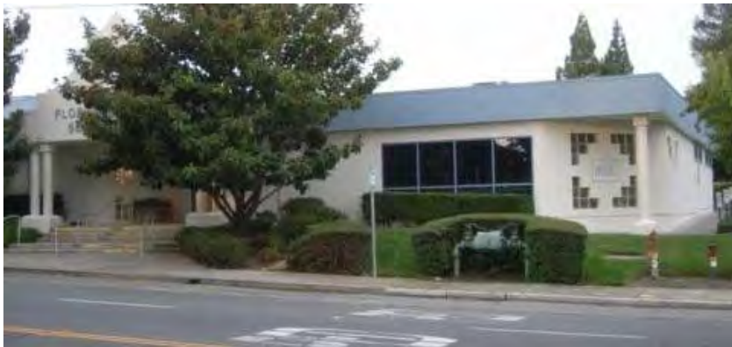
Figure 3: Florence Douglas Community Center
