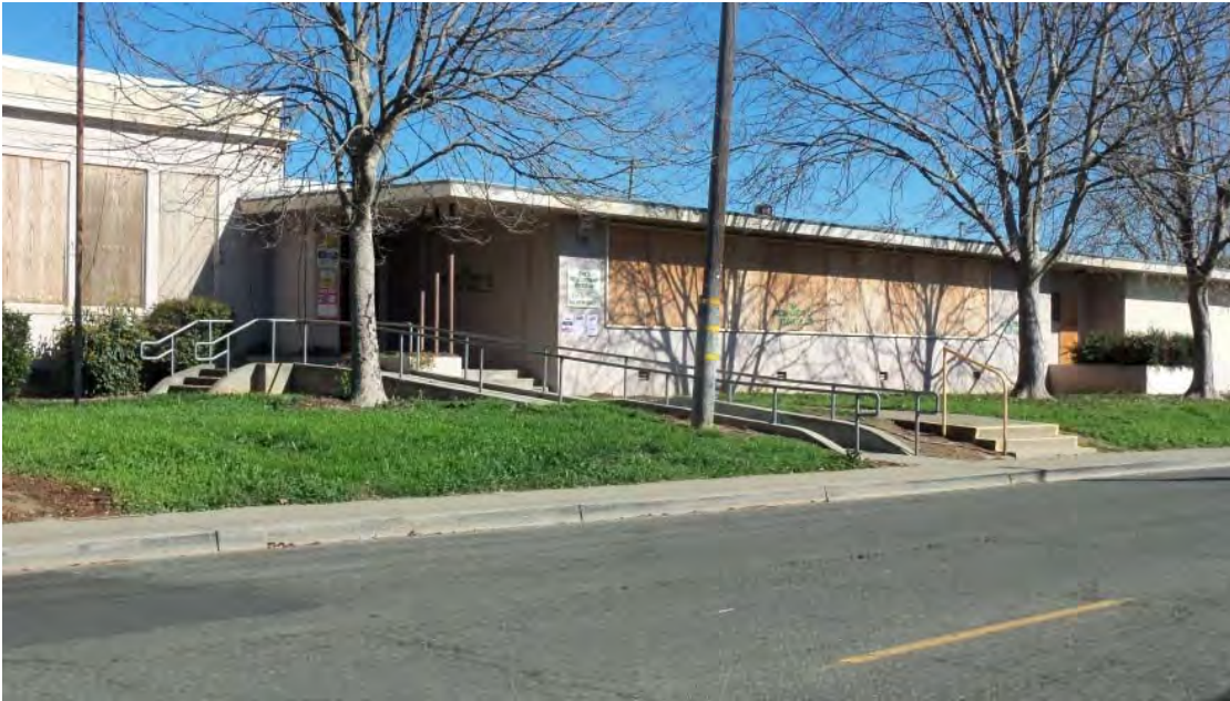
Figure 4: Vacant Grant School in South Vallejo
