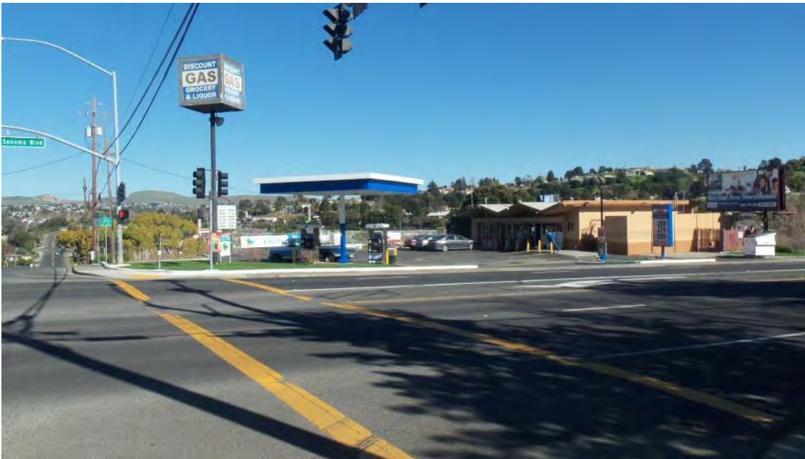
Figure 18: Key site to retrofit at corner of Magazine St. and Sonoma Blvd.
