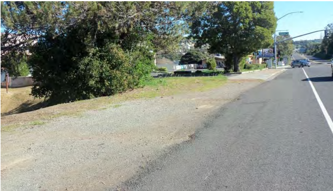
Figure 16: Gap in sidewalk on Sonoma Boulevard north of Magazine St.
