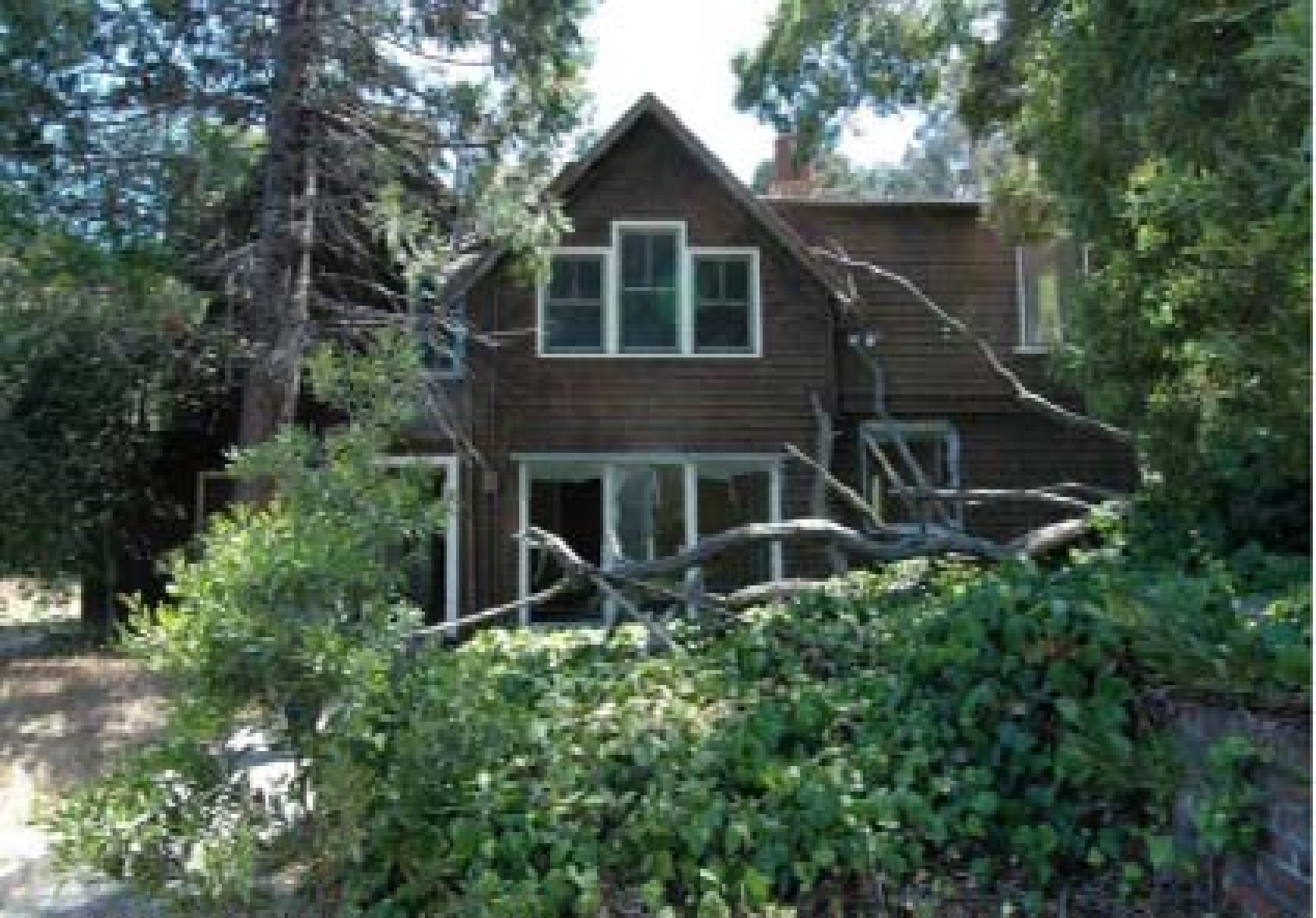
House, front (west) elevation. 1917 additions to left and right of central gable. © 2007.
