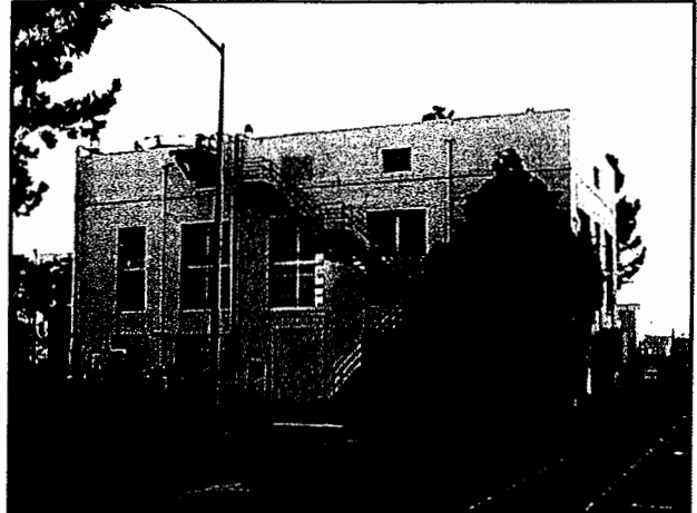
H – Other Infrastructure (Building H074)
