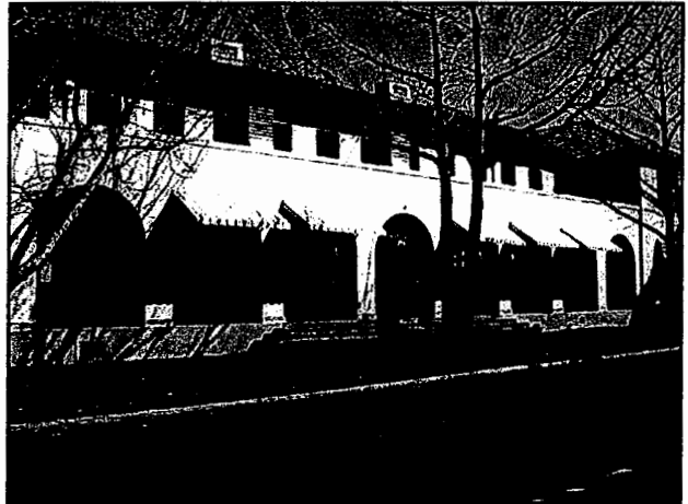
D – Barracks (Building 0459)
