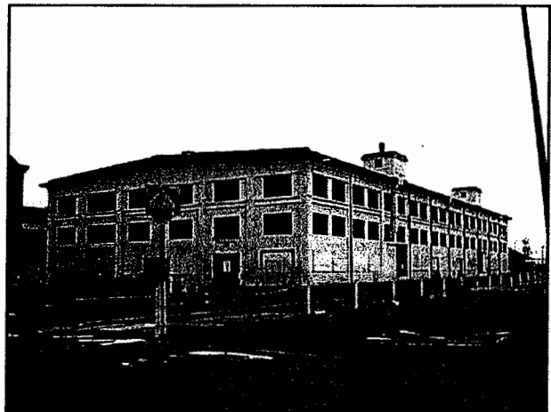
J – Masonry Industrial/ Ordinance Storage Or Warehouse (Building 0207)
