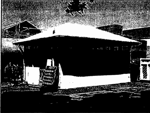
G – Latrine (Building 0077A)
