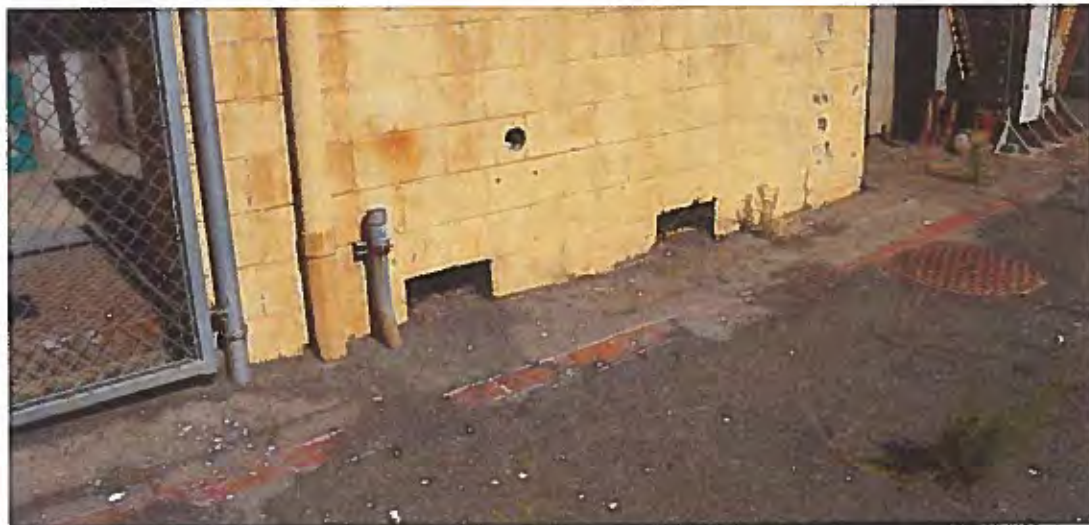
Image 9. South façade, typical drainage openings at the base of the wall.
