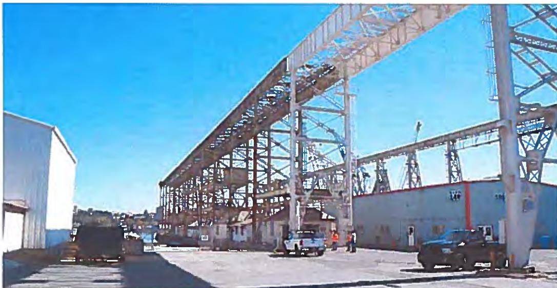
Image 1. Context view looking east at the subject dock with gantry crane with Building Ways #1 at the left.
