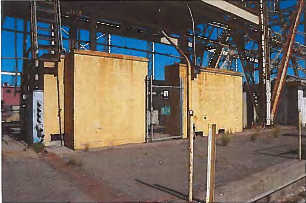
Image 3. South façade with central opening and chain link gate.
