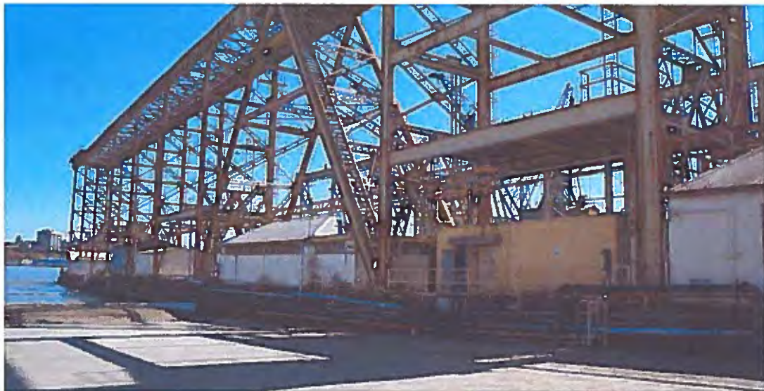
Image 2. Context view looking southeast from Building Ways #1 to the yellow subject building at the right of the image. Building 624 is located to the left of the subject building and Building 634 is partially visible at the far right. The end of the dock at Mare Island Strait is to the left.
