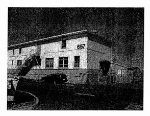
Building 657 is a two story reinforced concrete structure built in 1944. The building is rectangular in shape with the ground floor approximately 4 feet above grade. Steel stairs provide access into the building. A expansion joint was observed where the building was reportedly expanding in 1945. The roof is flat with a concrete overhang/eave. The building's area is approximately 7,000 square feet.
