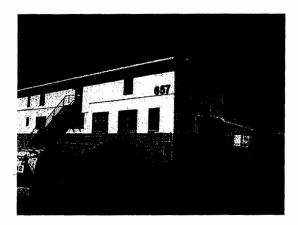
Building 657 is a two story reinforced concrete structure built in 1944. The building is rectangular in shape with the ground floor approximately 4 feet above grade. Steel stairs provide access into the building. A expansion joint was observed where the building was reportedly expanding in 1945. The roof is flat with a concrete overhang/eave. The building's area is approximately 7,000 square feet.
