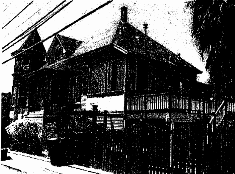
North east corner of residence. Inappropriate windows and building materials should be replaced. Thomas Cochrane photo, July 2005
